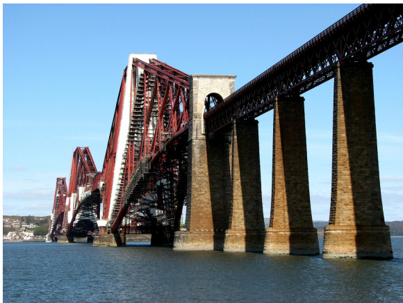
Figure: The Forth Rail Bridge
